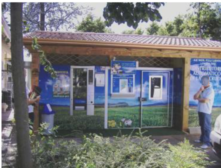
FIG. 10. Chalet-like facility on the outskirts of a park in a town in the Brescia province. 34
